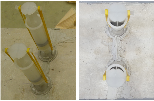
Fig. 4. Crack repairing process using epoxy
